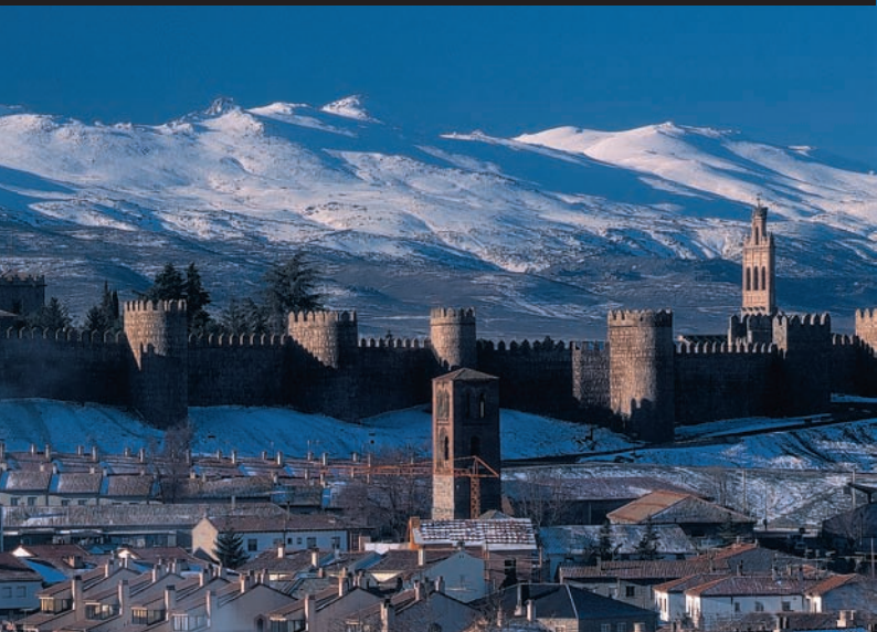
City walls. Avila
